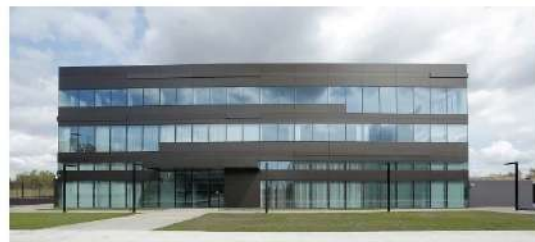
EnergyVille 2 building , open since May 2018
