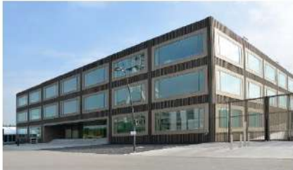
EnergyVille 1 building , open since April 2017
