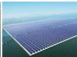
Assembly of connected floaters
