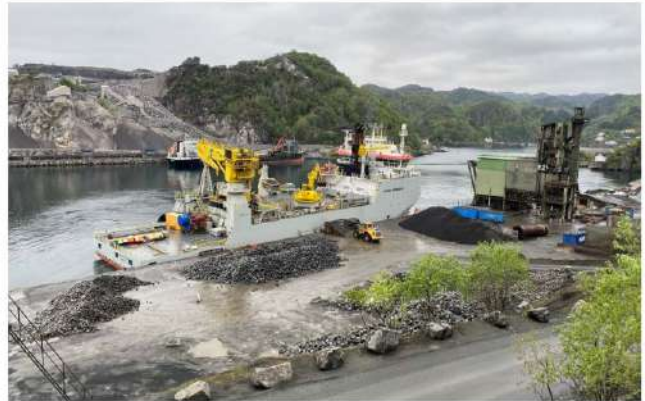
Doggerbank A OWF T&I scour protection
