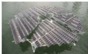
Assembly of connected floaters
