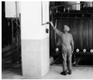
H 2 production plant in Rjukan, Norway 1929-1988, 167 MW 70 tons/day
